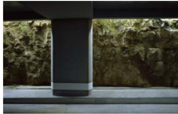
Paroi calcaire du parking / Limestone rock-face in the basement carpark
