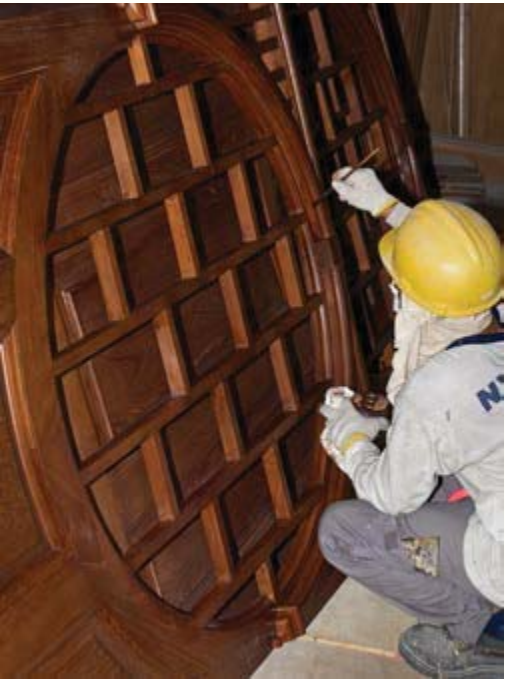
Restauration des lambris dans la Supreme Court Restoration of the timber paneling in the Supreme Court
