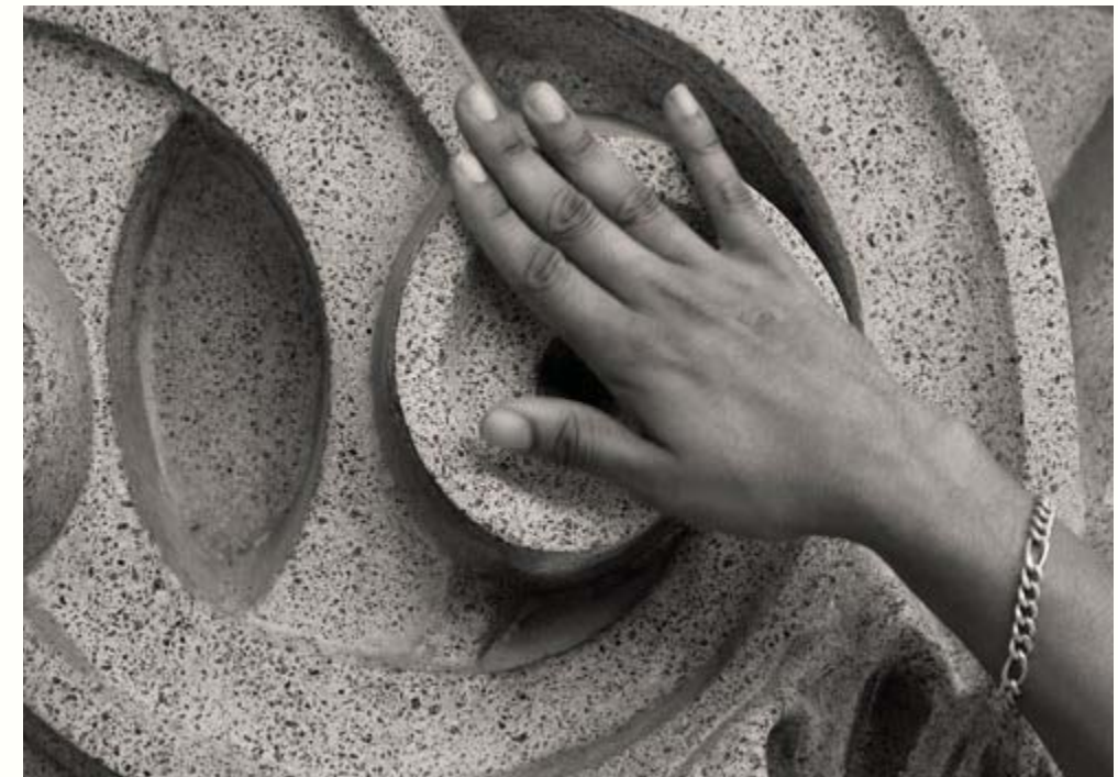
Détail de l'ornement de façade de la Supreme Court après nettoyage Assessment of the Shanghai plaster finish of the former Supreme Court façade after jet-cleaning
