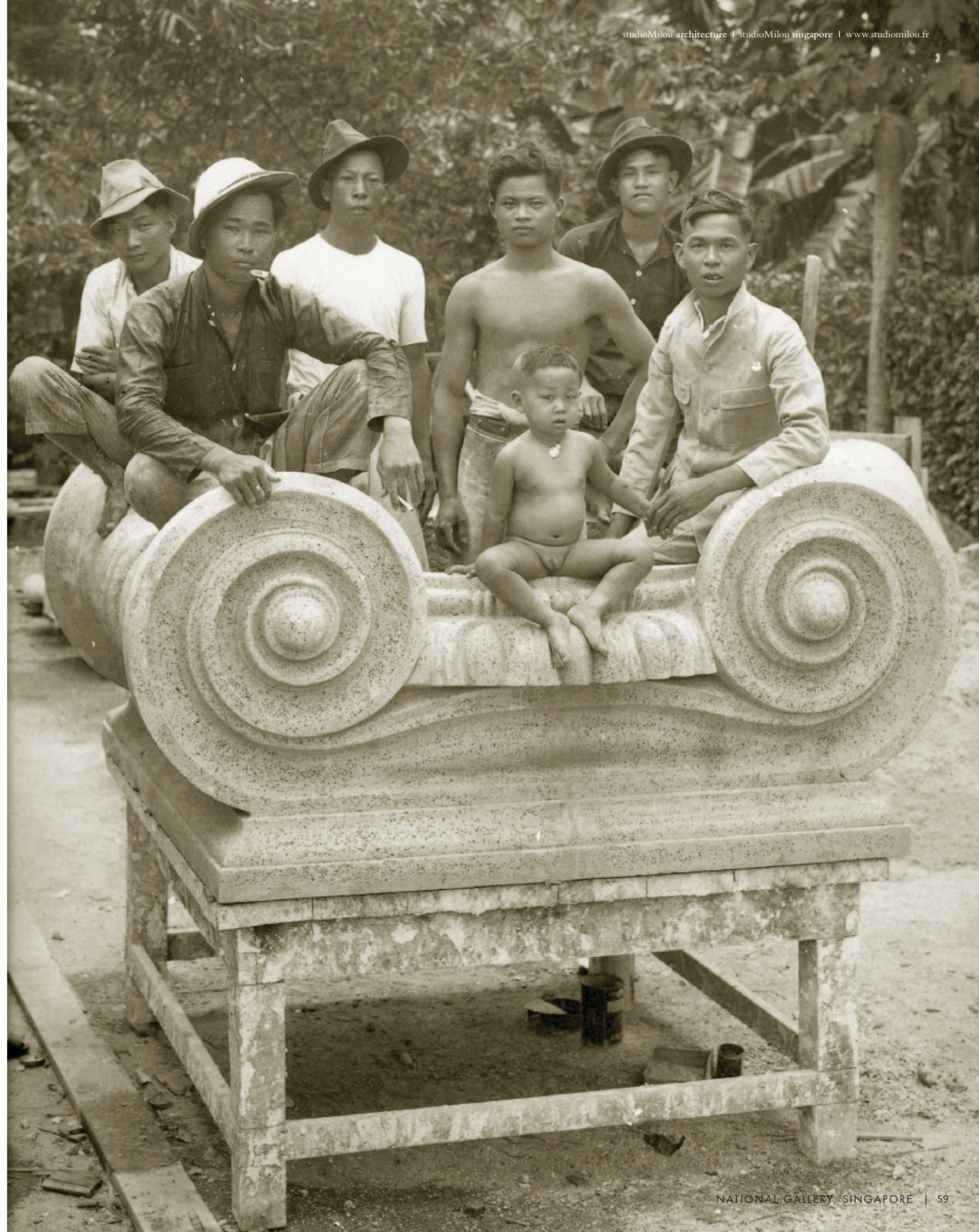
Element de façade prefabriqu  , atelier Nolli, Singapour, 1926 Prefabricated Ionic column capital of the former Supreme Court. atelier Nolli, Singapore, 1926
